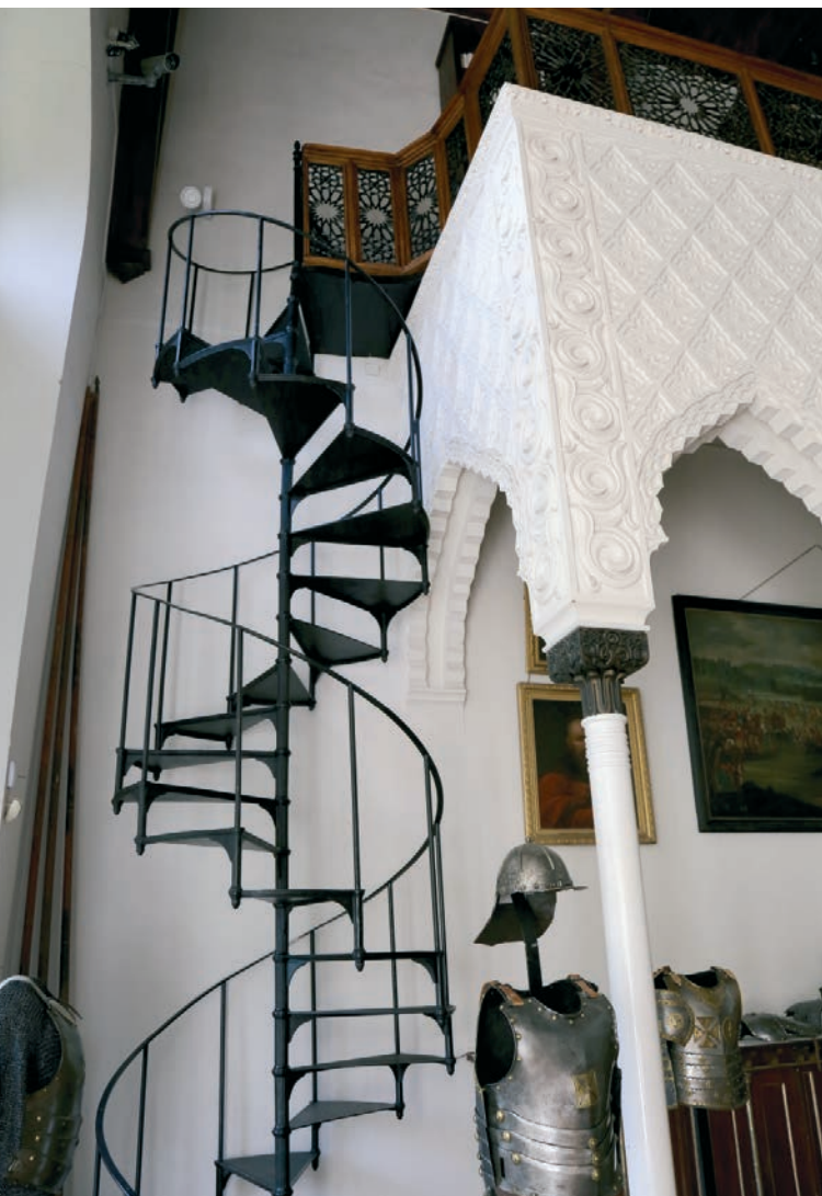
The Moorish Room – cast iron stairs leading to the gallery.
