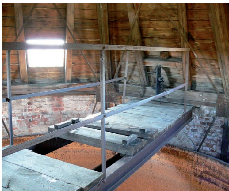
Upper platform above the tank
