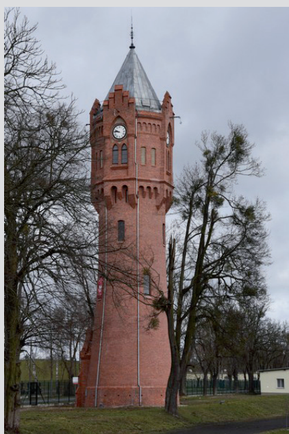
Southern elevation of the tower
