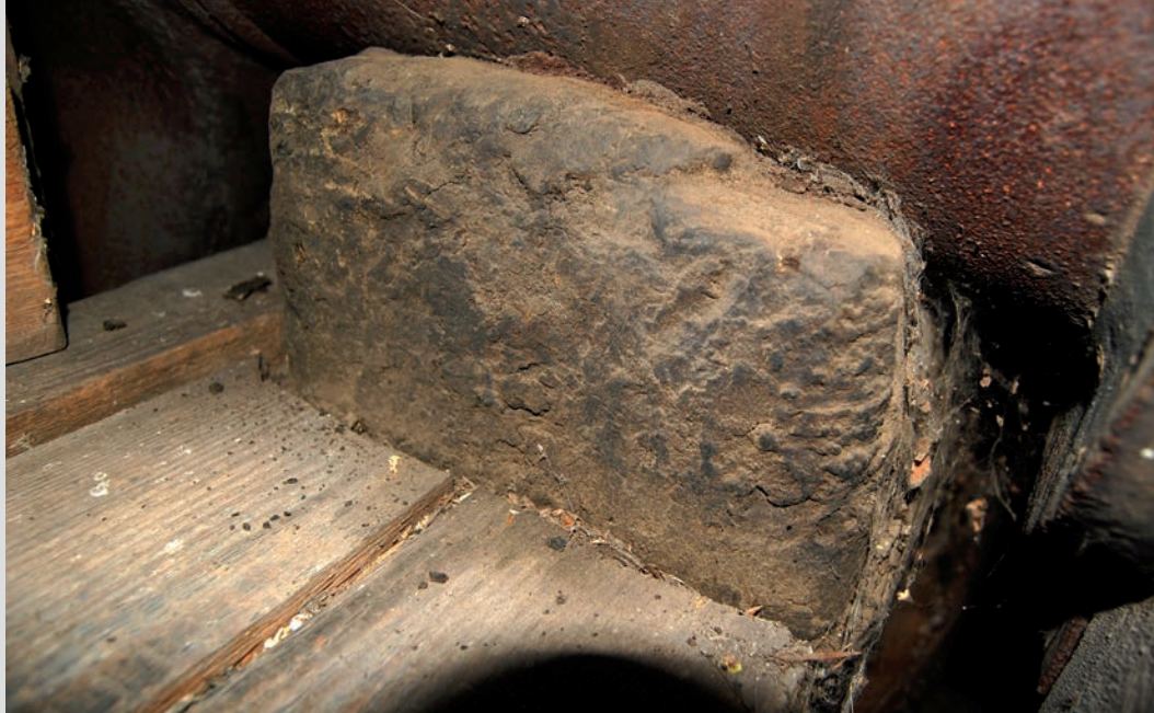
Wooden bearing from guaiac wood ( Guaiaacum officinale ) under the wing shaft head, photo: A. Pelczyk, 2019
