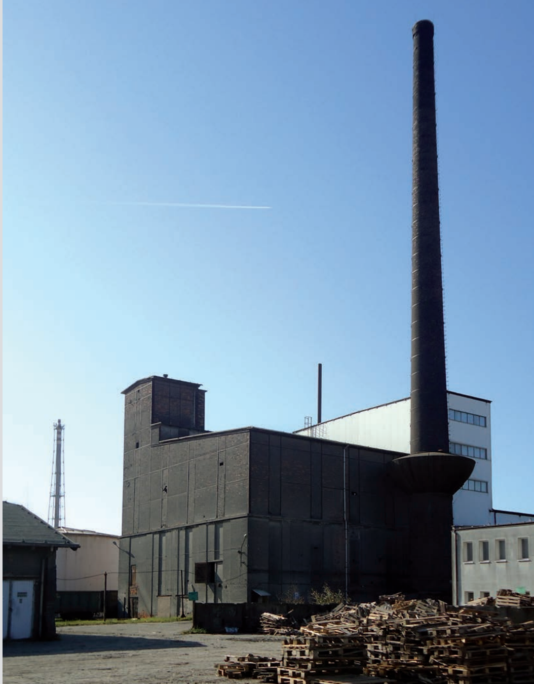
Chemical Plant in Luboń, boiler house with a chimney
